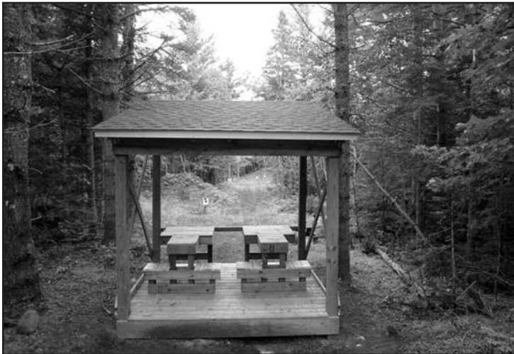
Tom Kehoe assisted by Mike Dudenas constructed a shooting shelter for the Club's shooting lane
